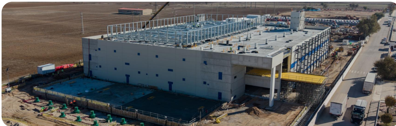
Alcalá Data Center, Madrid, Spain
