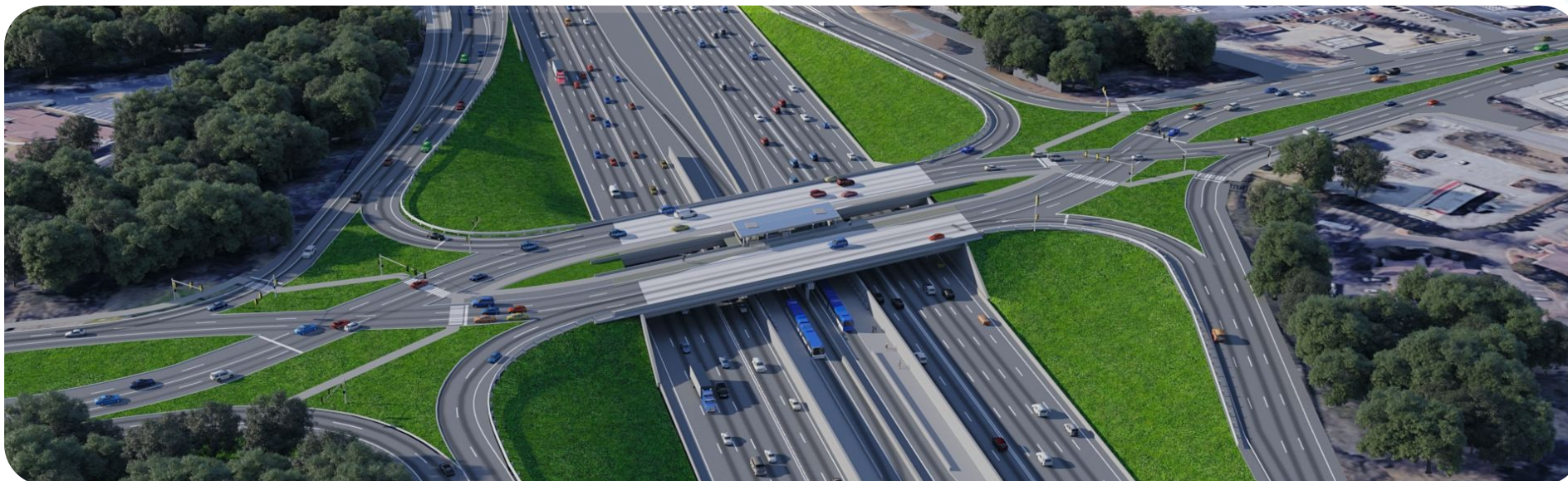
SR-400 Managed Lanes, Georgia, USA
