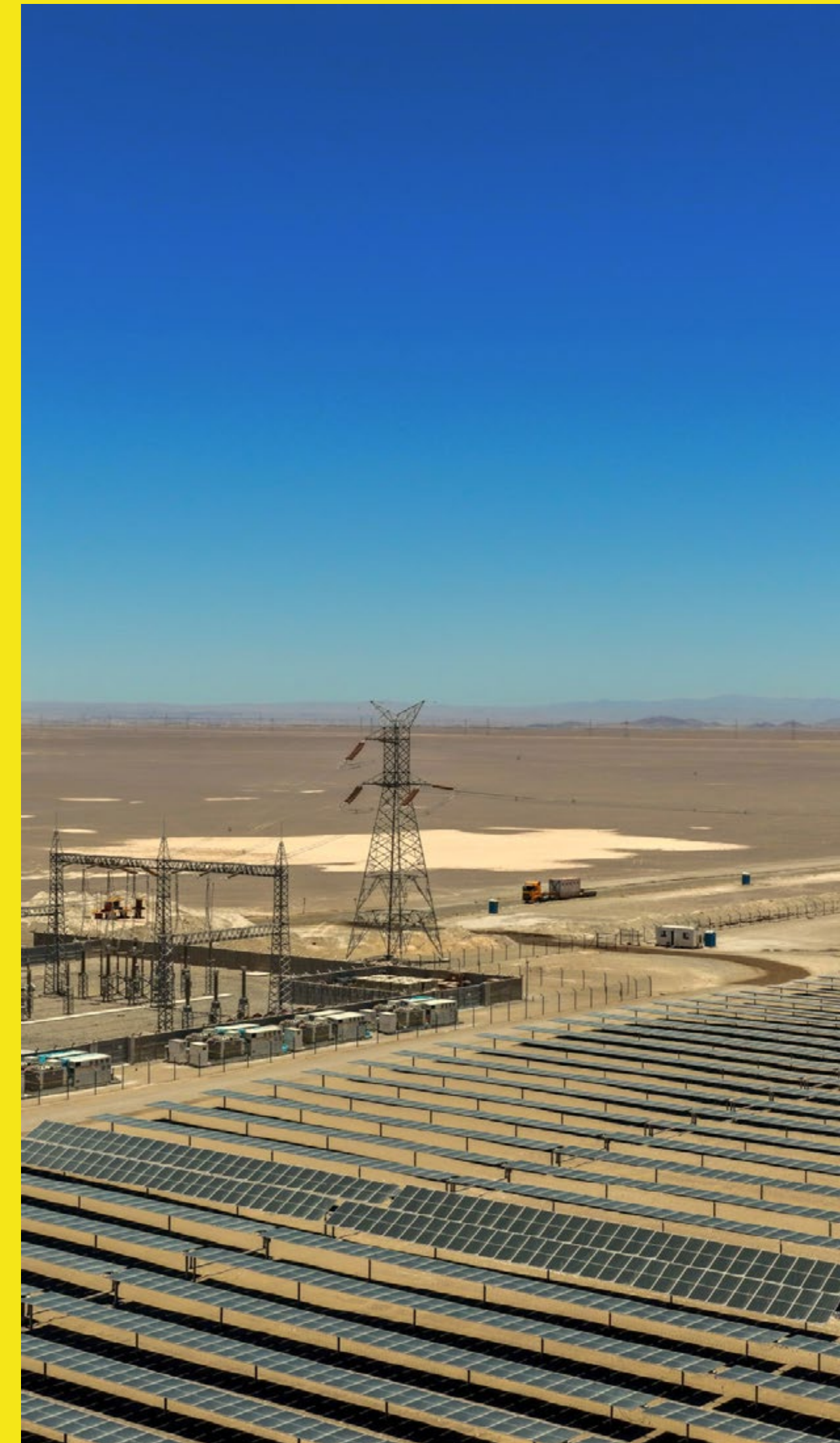
Elena 446 MW + 3.5 GWh hybrid plant, Chile
