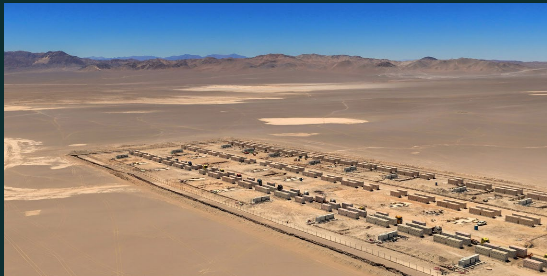
Elena 446 MW + 3.5 GWh hybrid plant, Chile
