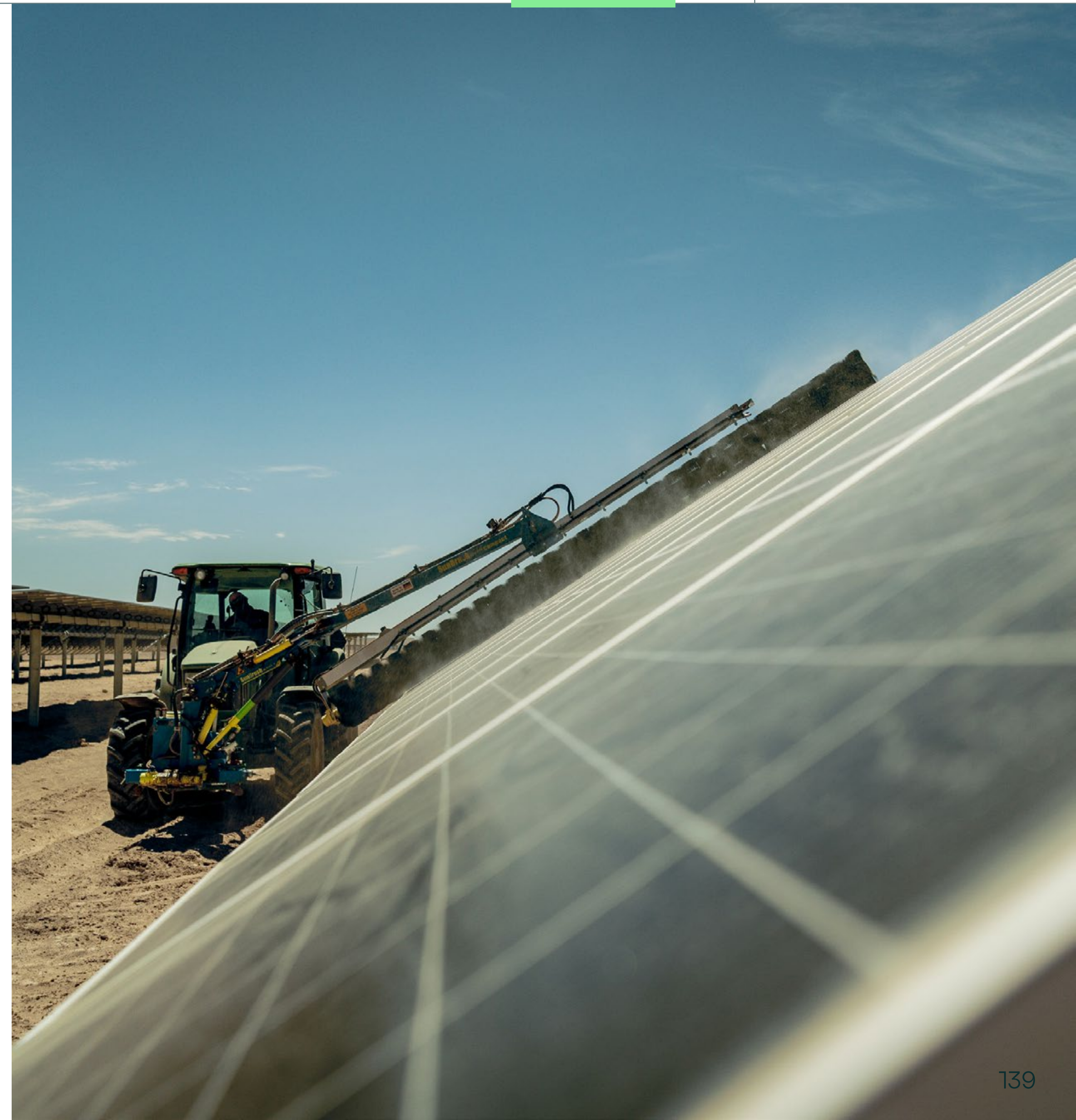
Cleaning of solar panels at the Quillagua PV plant, Chile
