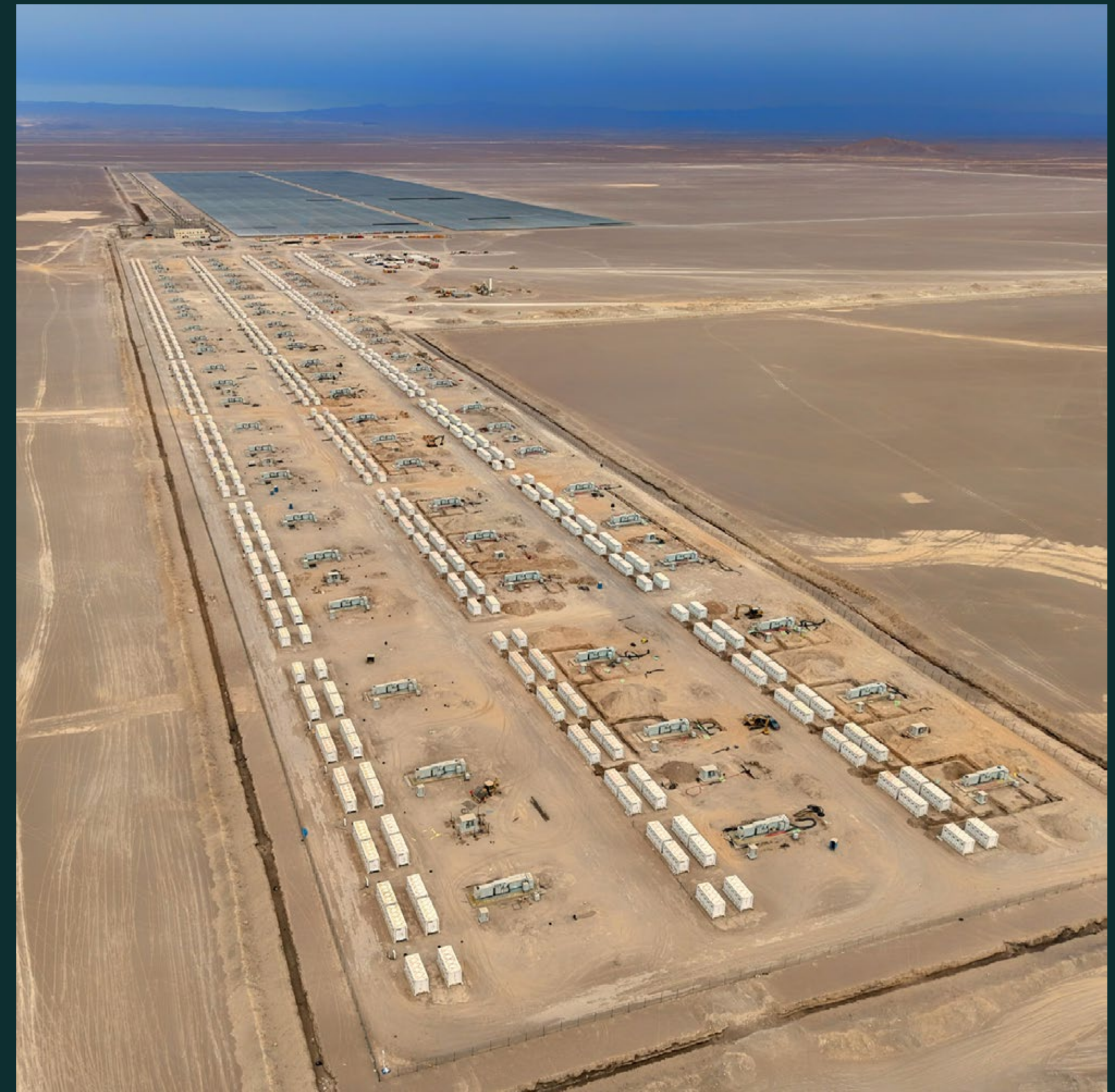
Elena 446 MW + 3,5 GWh hybrid plant, Chile
