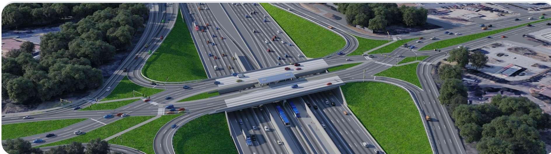
SR-400 Managed Lanes, Georgia, USA
