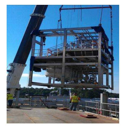
Eighteen super skids are being constructed in the "shop" on site and then transferred to the NFF building
