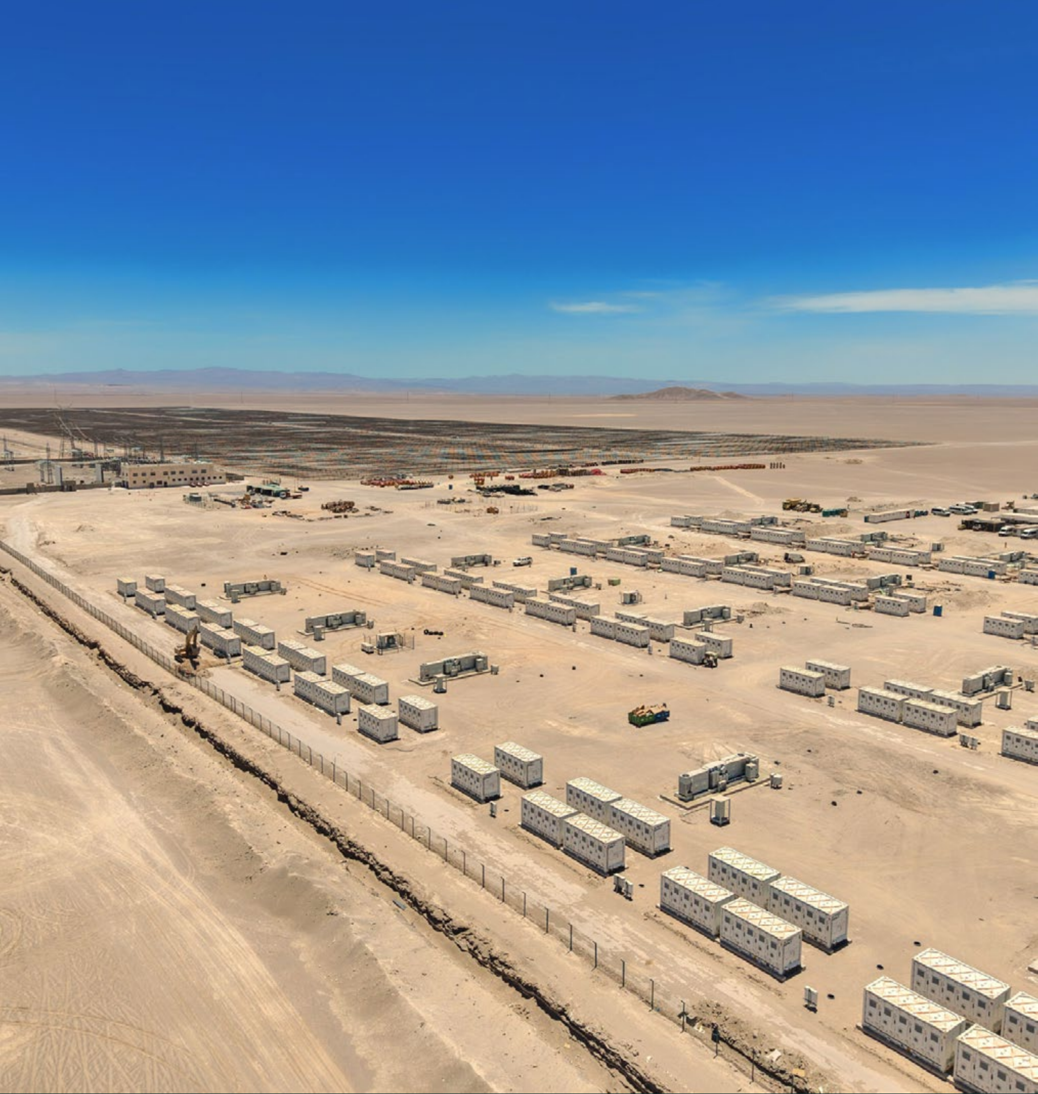
Elena 446 MW + 3.5 GWh hybrid plant, Chile
