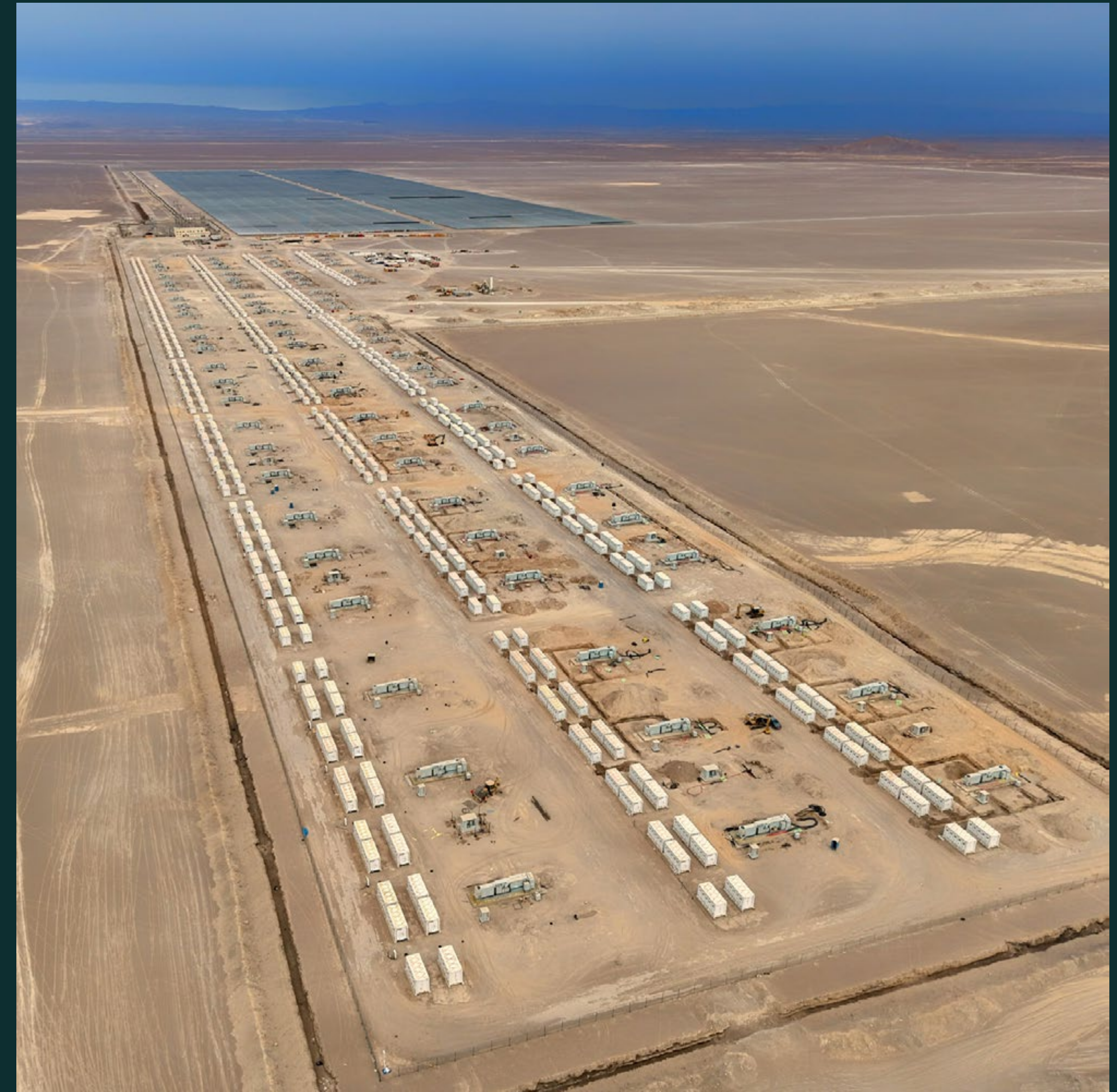
Elena 446 MW + 3.5 GWh hybrid plant, Chile
