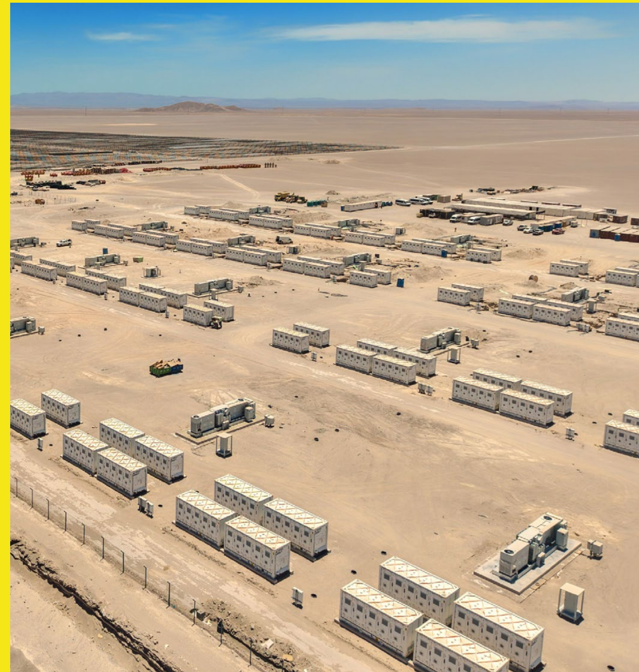
Elena 446 MW + 3.5 GWh hybrid plant, Chile
