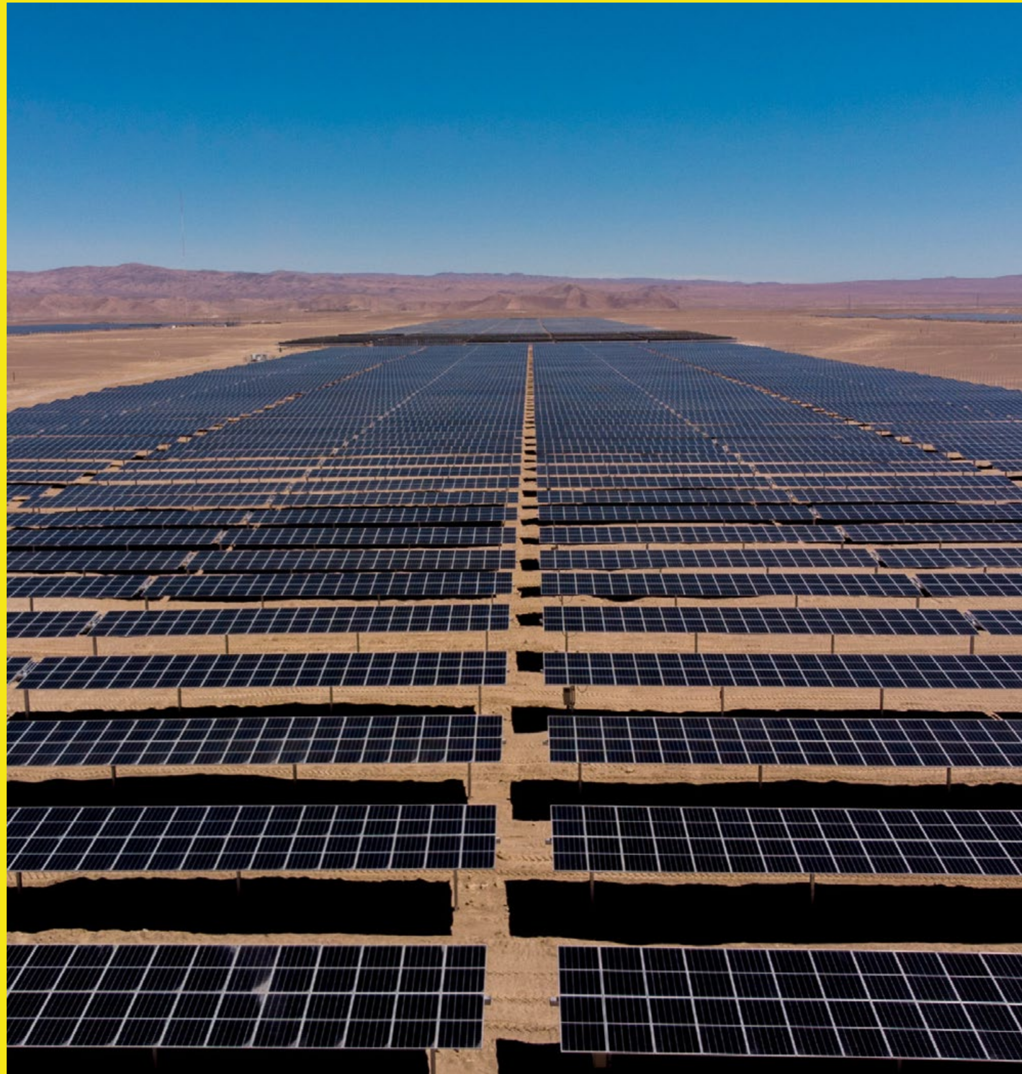
Quillagua 103 MW PV plant, Chile
