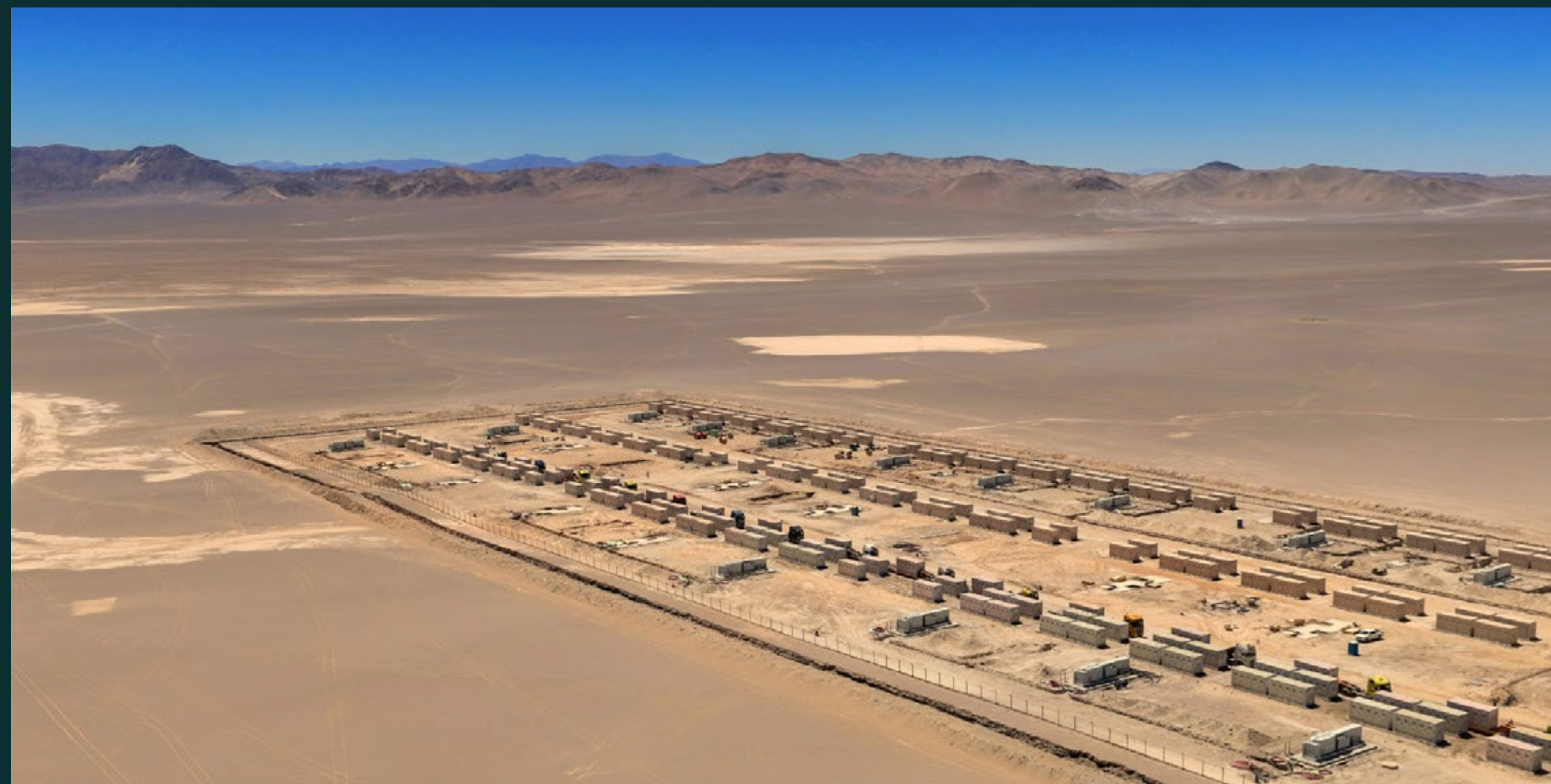
Elena 446 MW + 3.5 GWh hybrid plant, Chile
