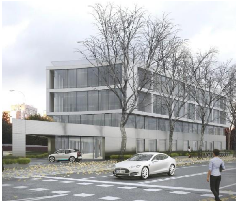
Photo: Árma. Computer graphic of the proposed design of Árma Paseo de La Habana (Fenwick Iribarren Architects).
